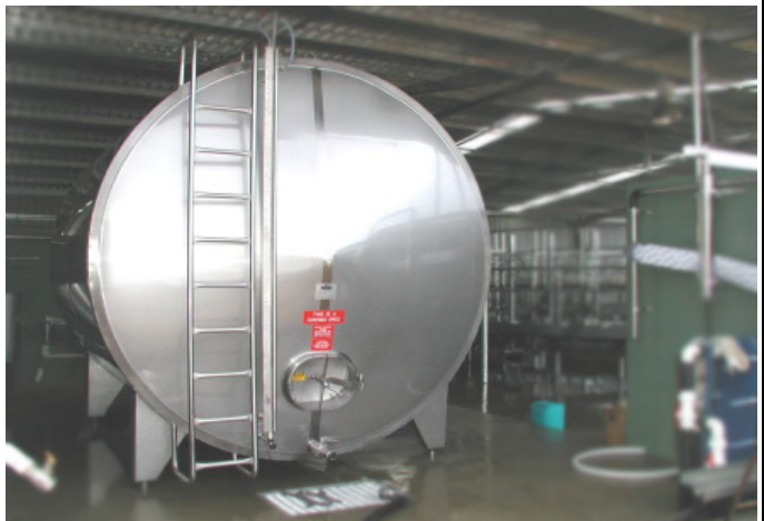
18,000L Horizontal Tank Installation.
